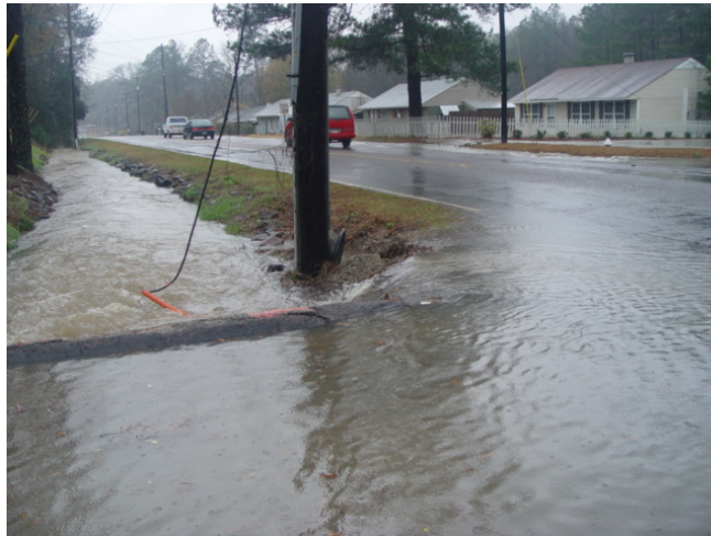
Figure 2: 2007- Flooding at Buena Vista and Mealing Avenue
