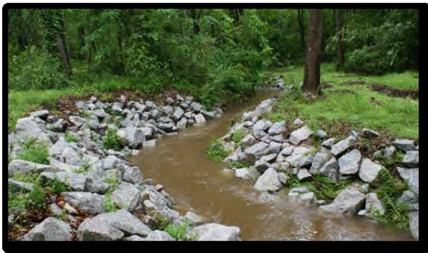
Figure 12: NA-PR-16 Bank stabilization in 2011
