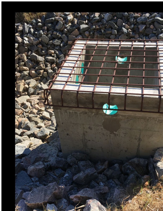
This outlet is clear and free of debris and vegetation.
