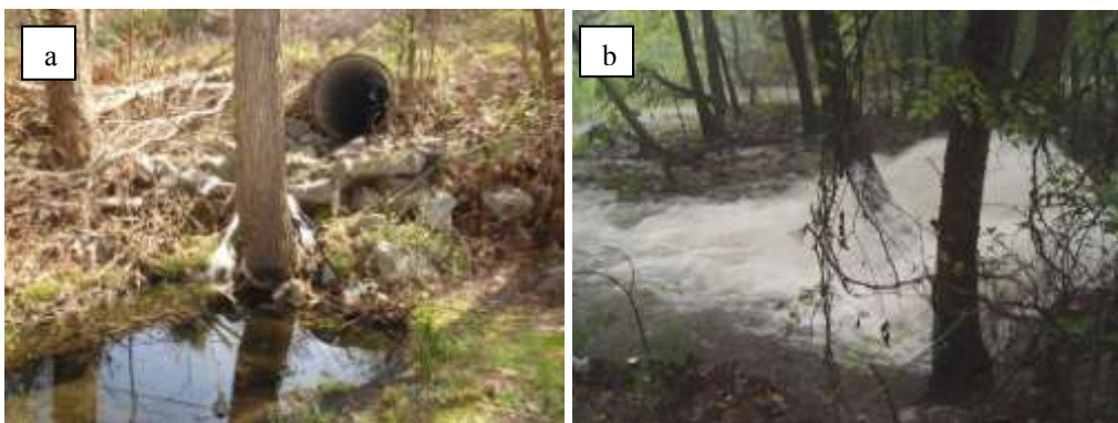
Figure 3. The stormwater runoff pipe into the eastern section of the restoration site during clear weather (a) and during a storm event (b).
