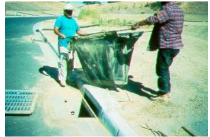
Geotextile curb inlet sediment barriers work well under low flow, low sediment conditions (see DrainGaurd above).
