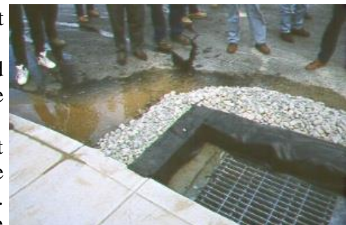
Block and gravel curb inlet sediment barrier.
