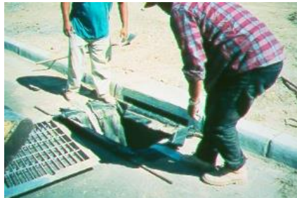
Geotextile curb inlet sediment barriers work well under low flow, low sediment conditions (see DrainGaurd above).
