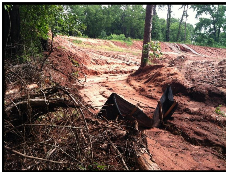
Silt fence should never to be used where concentrated flows occur.
