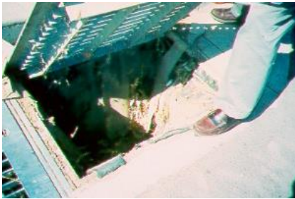
Geotextile curb inlet sediment barriers work well under low flow, low sediment conditions (see DrainGaurd above).
