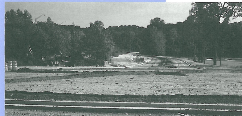
Construction of Riverside Boulevard
