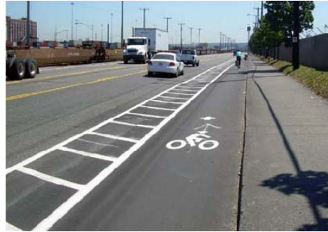
Seattle uses buffered bike lanes to protect cyclists from fast moving traffic.
