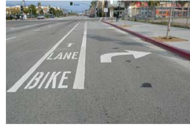
Continuing a bike lane straight while providing a right turn pocket reduces bicycle/motor vehicle conflicts.
