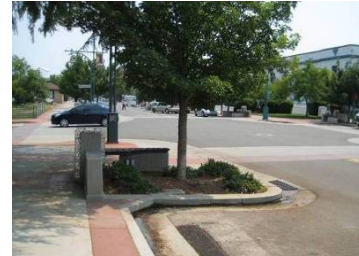
Curb bulb-outs can be a good location for pedestrian amenities and street trees.
