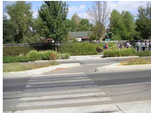
An offset crossing forces pedestrians to turn and face the traffic they are about to cross.
