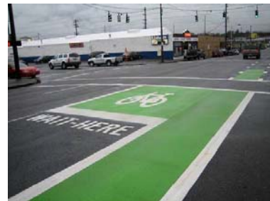
Bike boxes have been installed at several intersections in Portland, Oregon where right-turning motorists conflict with through bicyclists.
