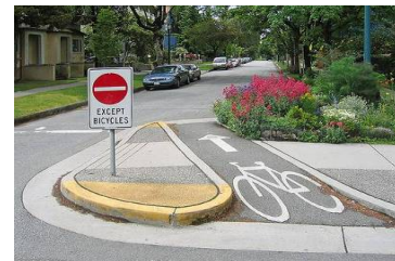
Choker entrances can be used to minimize vehicle turns onto a boulevard.
