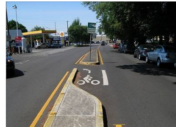
This bike-only left turn pocket guides cyclists along a popular bike route.
