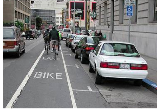
This bike lane provides parking “T”s to minimize the risk of “dooring”.
