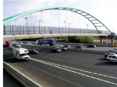
Type 4 Grade-Separated Overcrossing
