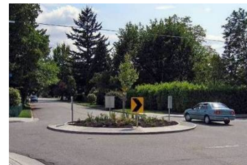
Roundabouts require that both bicyclists and motorist slow down and watch for conflicts.
