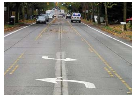
This road was re-striped to convert four vehicle travel lanes into three travel lanes with bike lanes.
