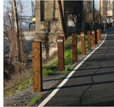
Post and Wire Fence
