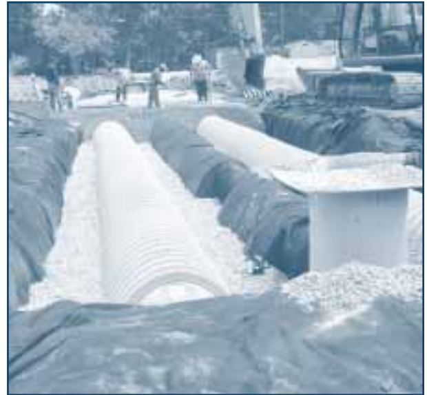
Workers covering the storm tech system
