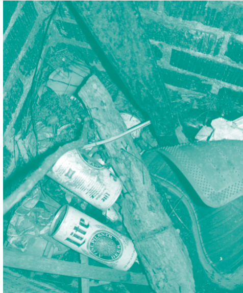
North Augusta Storm Drain Inspection
