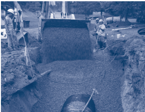
City workers repairing Bolin Court storm sewer line.
