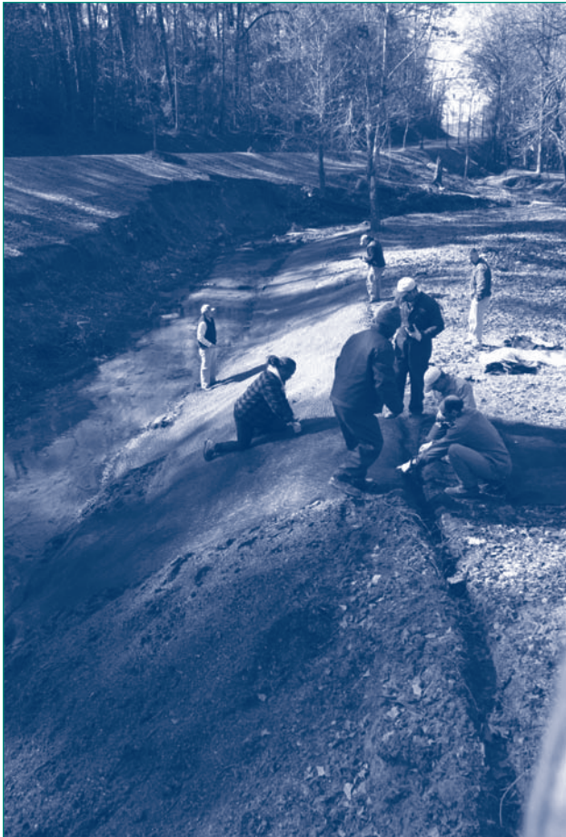
Slope repair product testing along Greenway Trail
