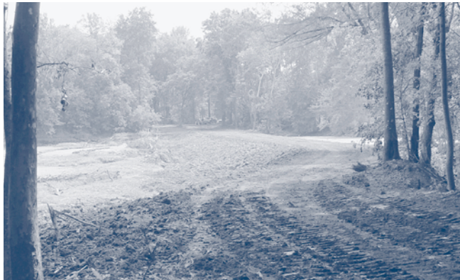
East pond dam under construction.
