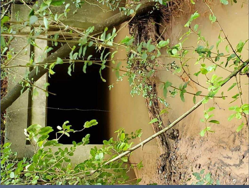
Brandenburg Detention Area – Crossing under I-20 Exit 5 (to Pole Branch)
