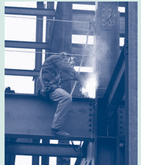
Municipal Center construction is well underway and on schedule.
