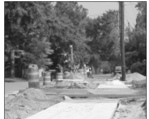
Construction on Brookside Drive nears completion.
