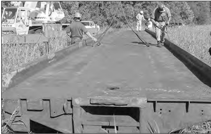
Donated by TTX Hamburg Division, this 90-foot flatbed railcar will soon serve another useful purpose as a bridge over Crystal Creek as part of the Greenway Riverfront Extension.
