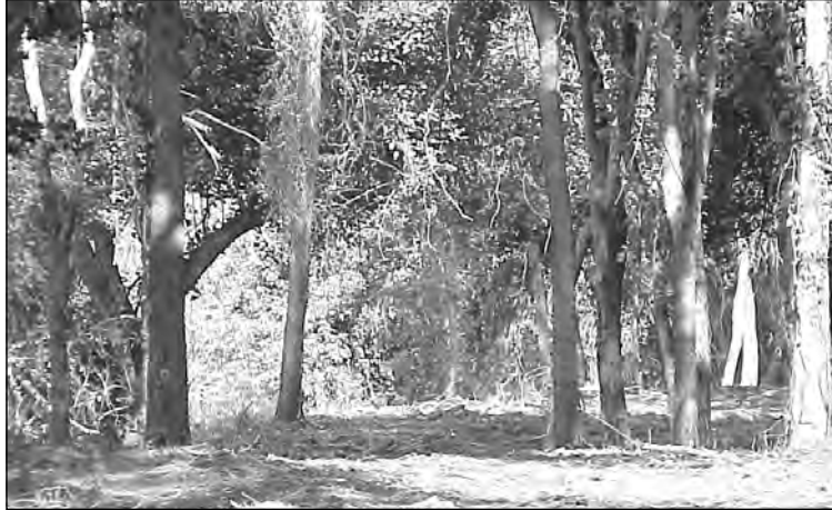
Riverfront Park and Greenway clearing in preparation for construction.
