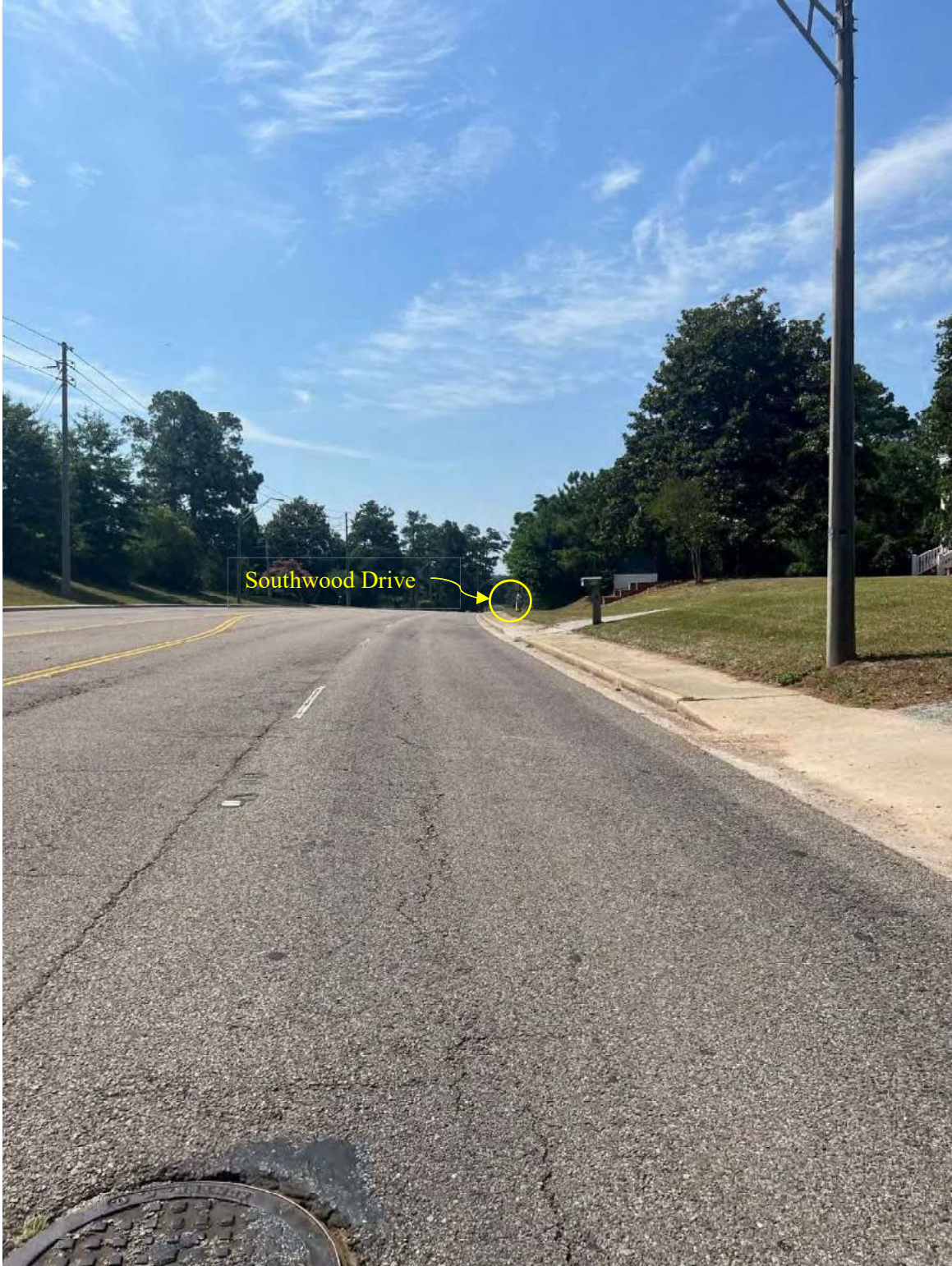
Approaching sight distance from the north.
