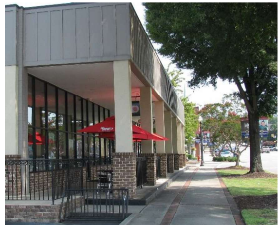
▼ After photo of renovated building
