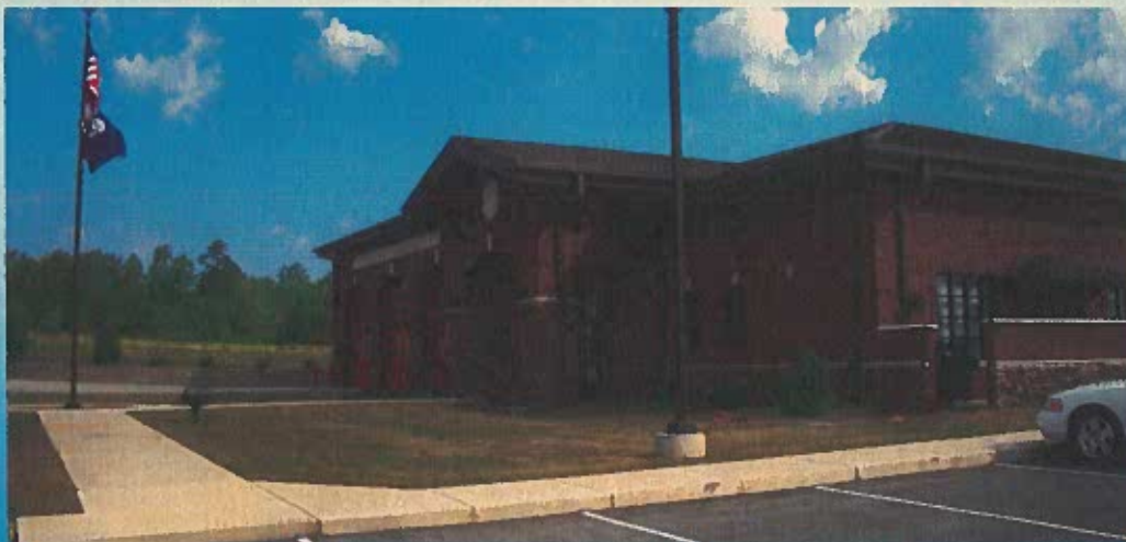
Station 3 692 Belvedere Clearwater Road
