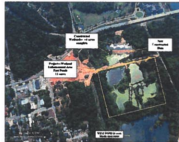
Fig. 3. Aerial view of 30 acres of wetland and upland along Savannah River that is being retrofitted.
