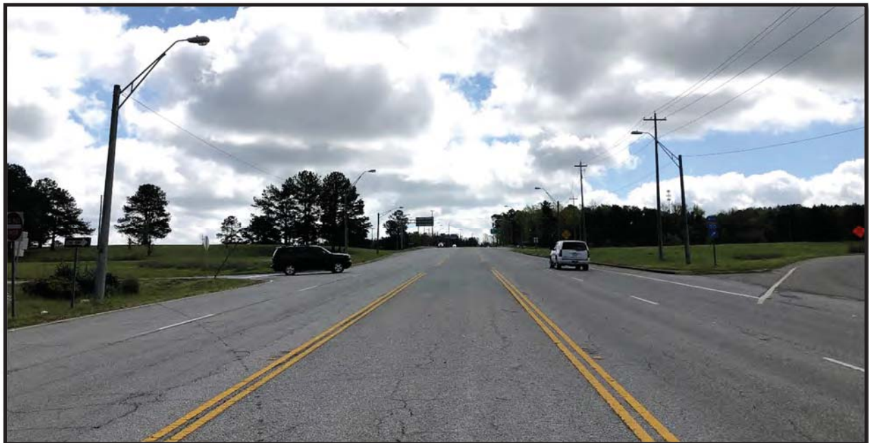
West Martintown Road looking south (uphill) at I-20 Westbound Ramps
