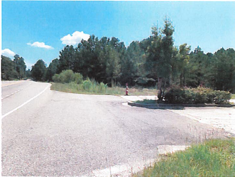
Figure 1: Entry view looking south along Five Notch Rd.
