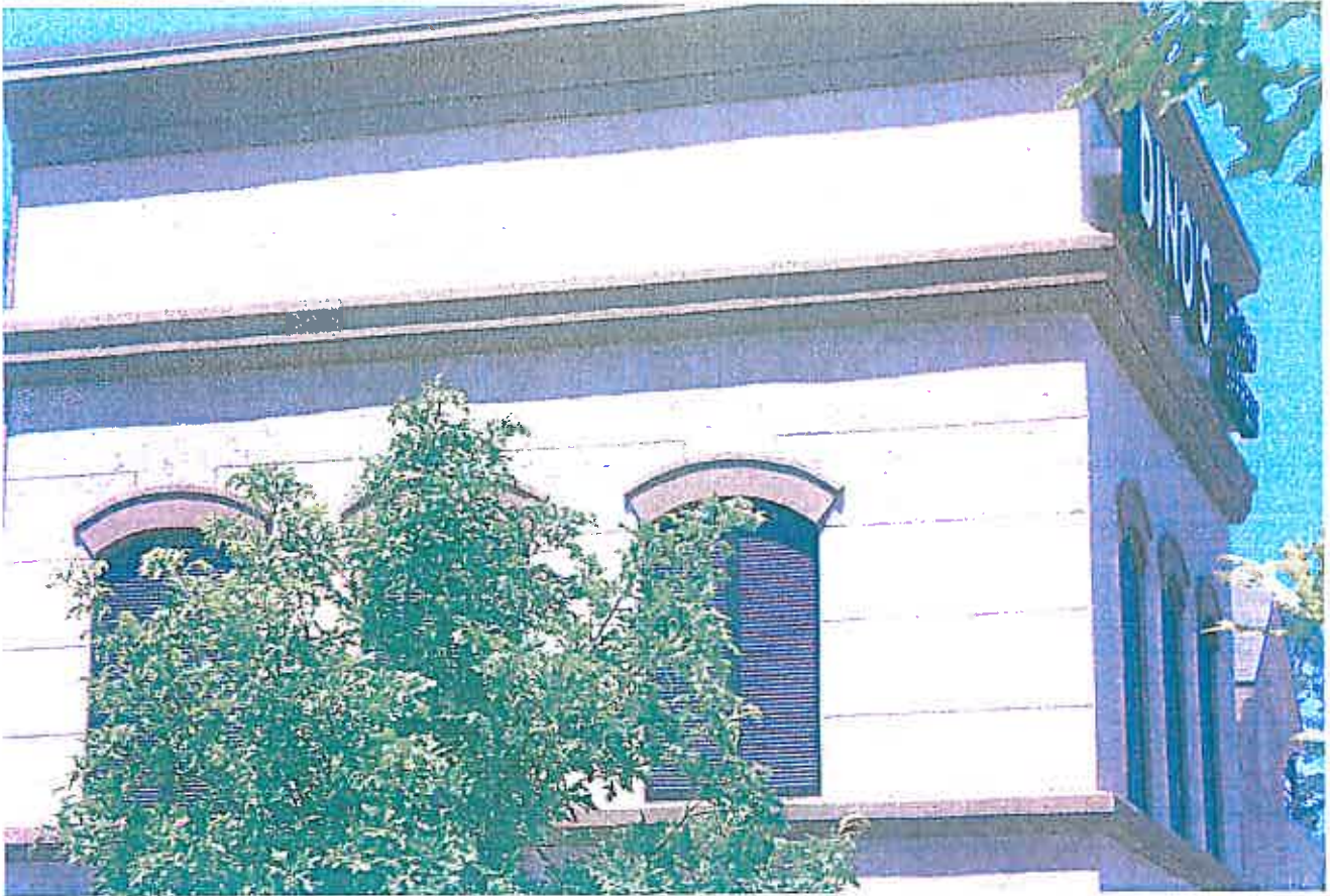
Example of Stucco "Texture" Finish
