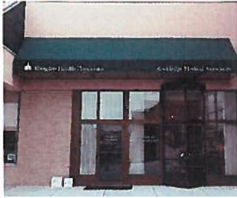
Figure 2: Awning & Awning Sign
