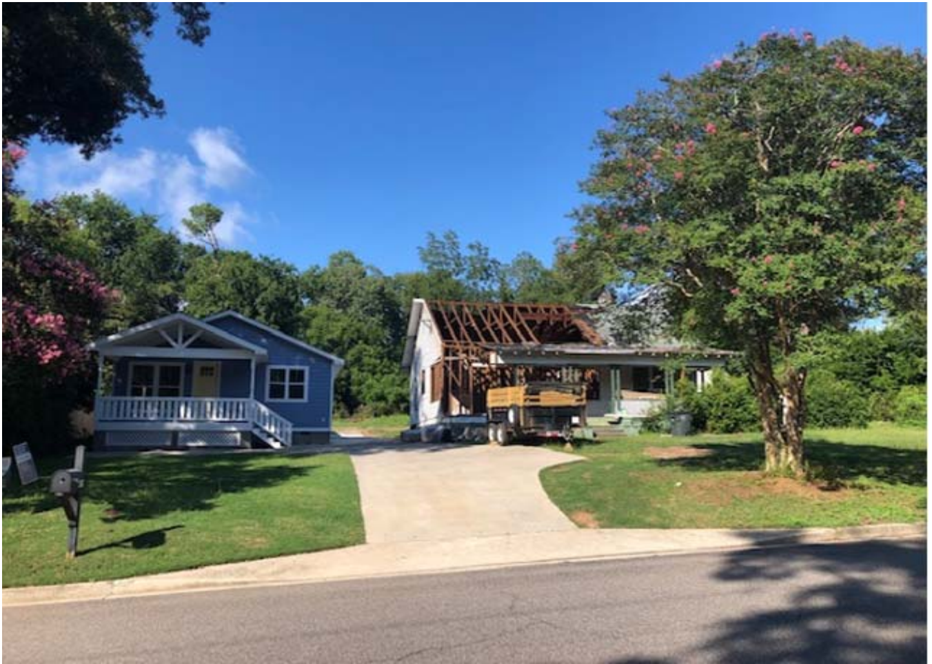
Existing shared driveway for 419 and 417 W. Woodlawn Ave.
