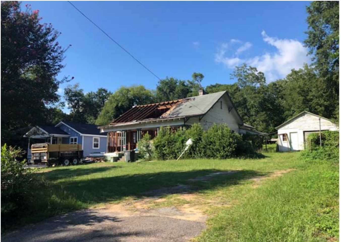
Existing driveway access to 417 W. Woodlawn Ave
