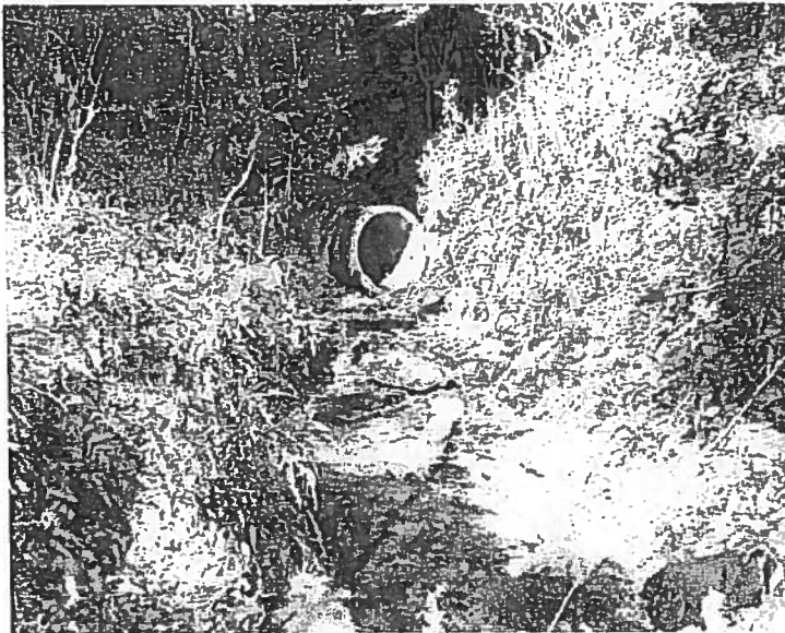
Figure 2. The location of 52-inch concrete pipes which allow drainage from surrounding neighborhood to pass under the Greenway and through this property.
