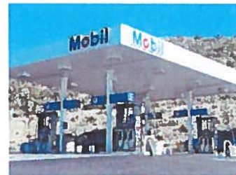
Figure 3: Canopy and Canopy Sign
