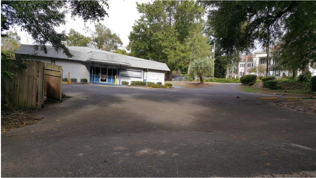
Figure 8: View from site from Carolina Ave. park area
