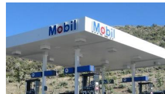
Figure 3: Canopy and Canopy Sign
