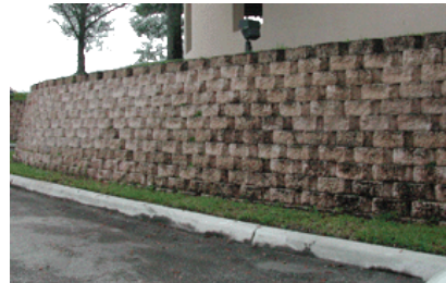
FIGURE 3-13 TEXTURED BLOCK RETAINING WALL
