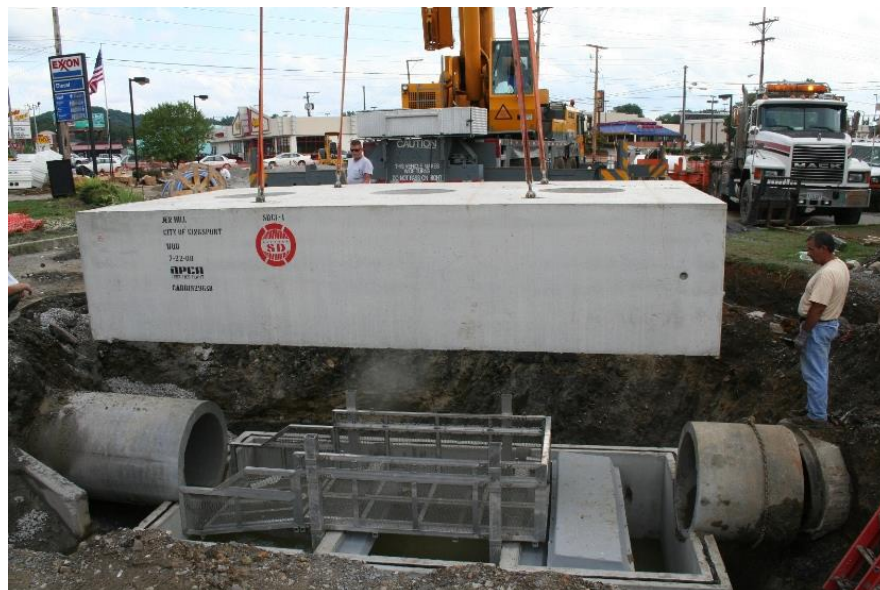
Illustration 1: Suntree Device being installed City of Kingsport, TN
